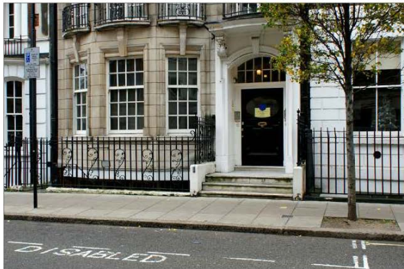
PHOTOGRAPH OF EXISTING FRONT ENTRANCE
