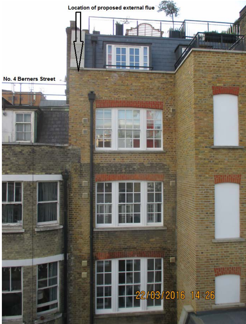
Photograph 1- Rear elevation of 5 Berners Street
